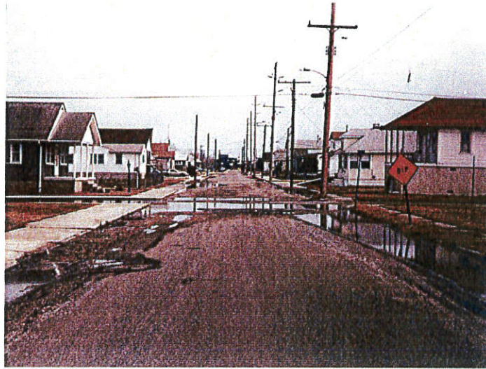
Pine Avenue at Avenue J 1990 Pre-constriction Photograph
